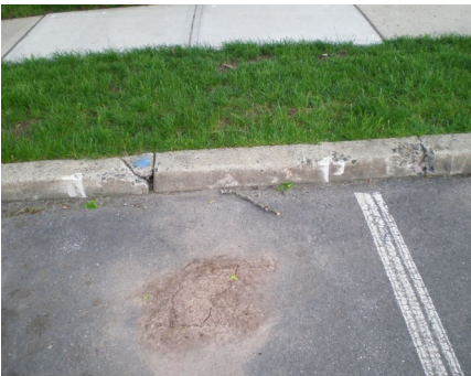
Deteriorating concrete curbs were replaced
