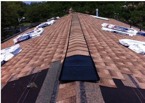
New shingles being installed
