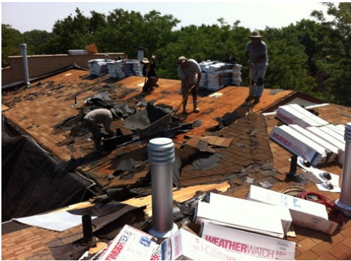
Removal of old shingles
